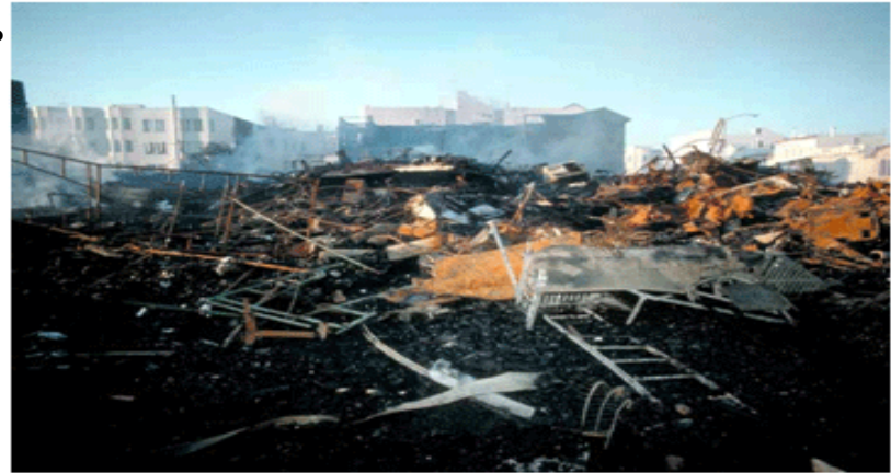
SF Marina district, Loma Prieta earthquake: Homes built on liquefied soil
